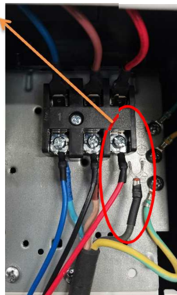
ODU terminal block wiring
